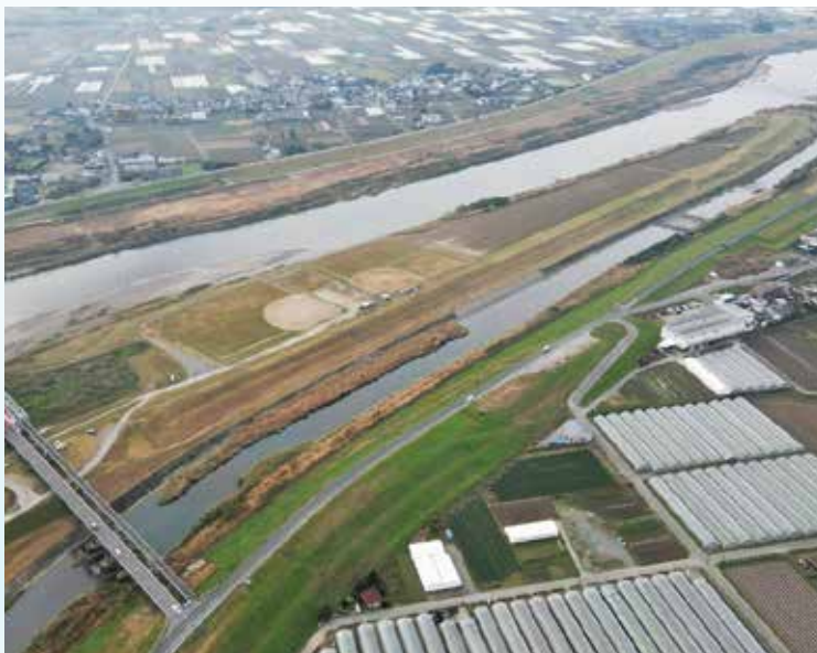
▲小石原川導流堤
